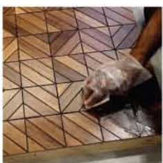
Step-9: Fill epoxy grout material
