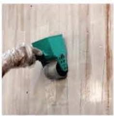
Step-4: Apply glue to liner material
